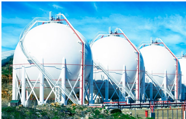
Figure 5: Insulated spheres for liquid storage of gaseous materials
